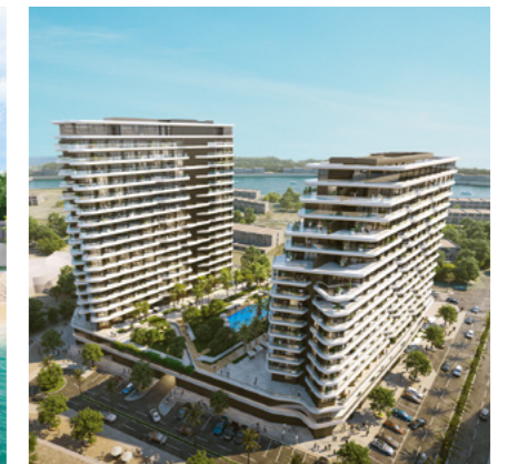
BAYVIEWS HAYAT ISLAND, MINA AL ARAB, RAS AL KHAIMAH Residential Buildings
