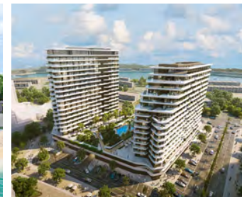
Bay Views Hayat Island, Mina Residential Buildings
